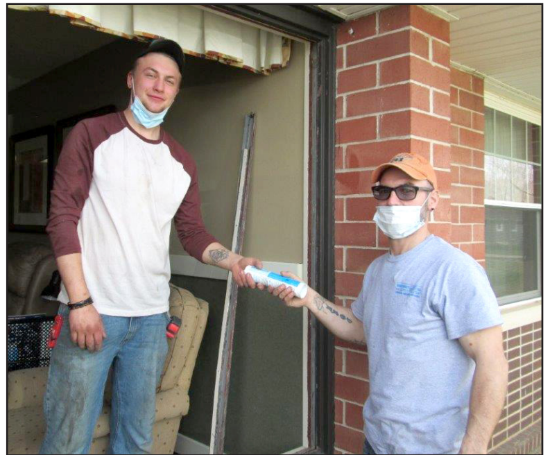
Northwest Glass Company guys put in a new window for us.
